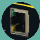
IEC 61850 server Ethernet port
